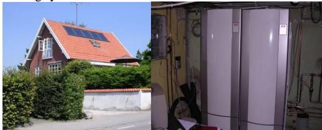
Fig. 4. Demonstration house with collectors on the roof and the solar tank and technical unit in the basement.
