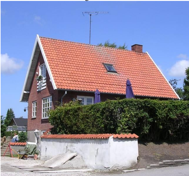
Fig. 1. Demonstration house from the south before installation of the solar heating system.
